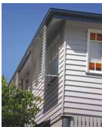
Figure 9 An example of how effectively the vertical screen shades the window from low-angled sun.
