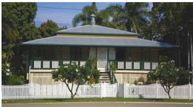
Figure 1 Full wrap-around verandah (Photo: TCC).
